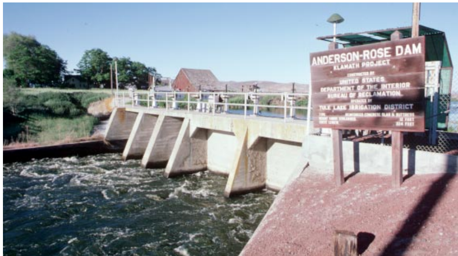
USBR’s Anderson-Rose Dam is located on the Lost River in Oregon, just north of the stateline. This Klamath Project facility diverts water to serve irrigation needs on the bed of the former Tule Lake in California and Oregon.
